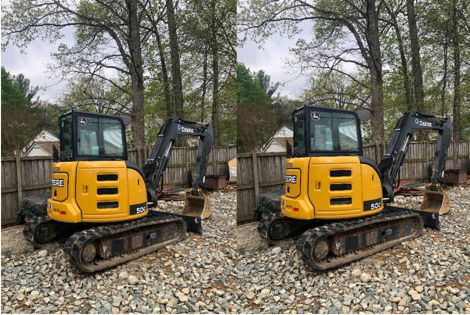
April 25, 2020: Construction of Retaining Wall on Lee Chapel Rd in Burke VA
