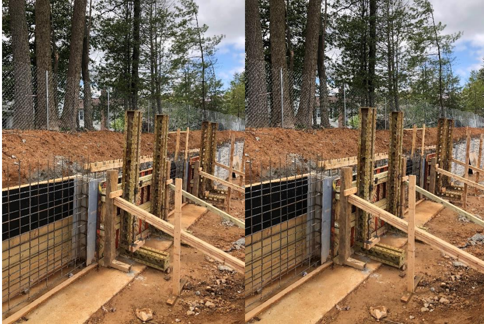
April 18, 2020: Construction of Retaining Wall on Lee Chapel Rd in Burke VA
